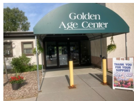
Welcoming Front Entrance
