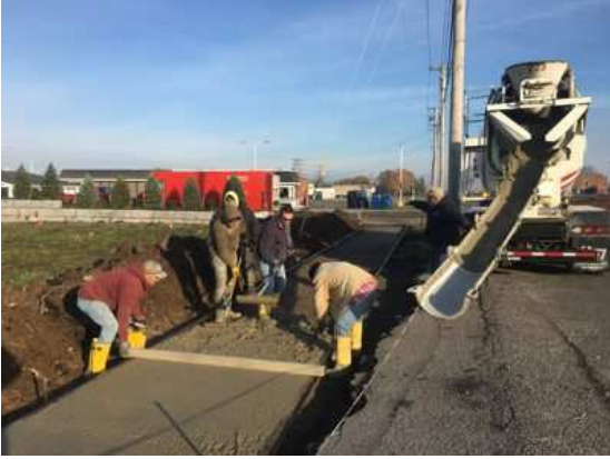
Sidewalk on Baseline Road.
